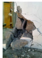
Pillar disintegration
